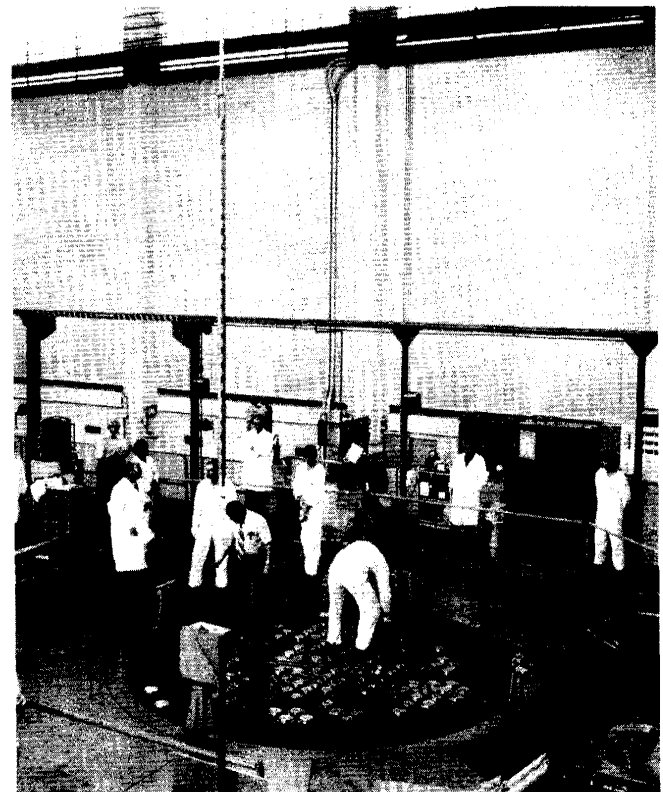
The top of the NRU reactor in Canada, where fuel rods are being tested under LOCA conditions, is shown above. The test train containing 32 rods, each 12 feet long, is being lowered into the in-pile test loop.
