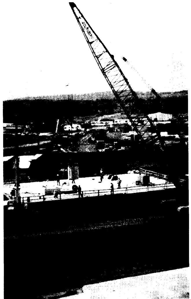
Removal from waste storage of a liner from the first stage of EPICOR-II for shipment to the Battelle Columbus Laboratories for examination.
